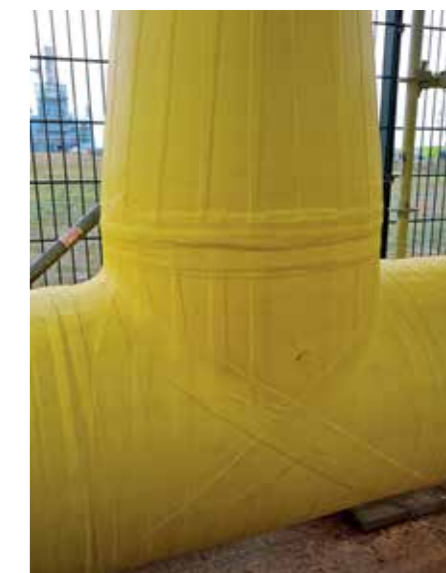
Coating pipes on site can avoid expensive, lengthy shutdowns
